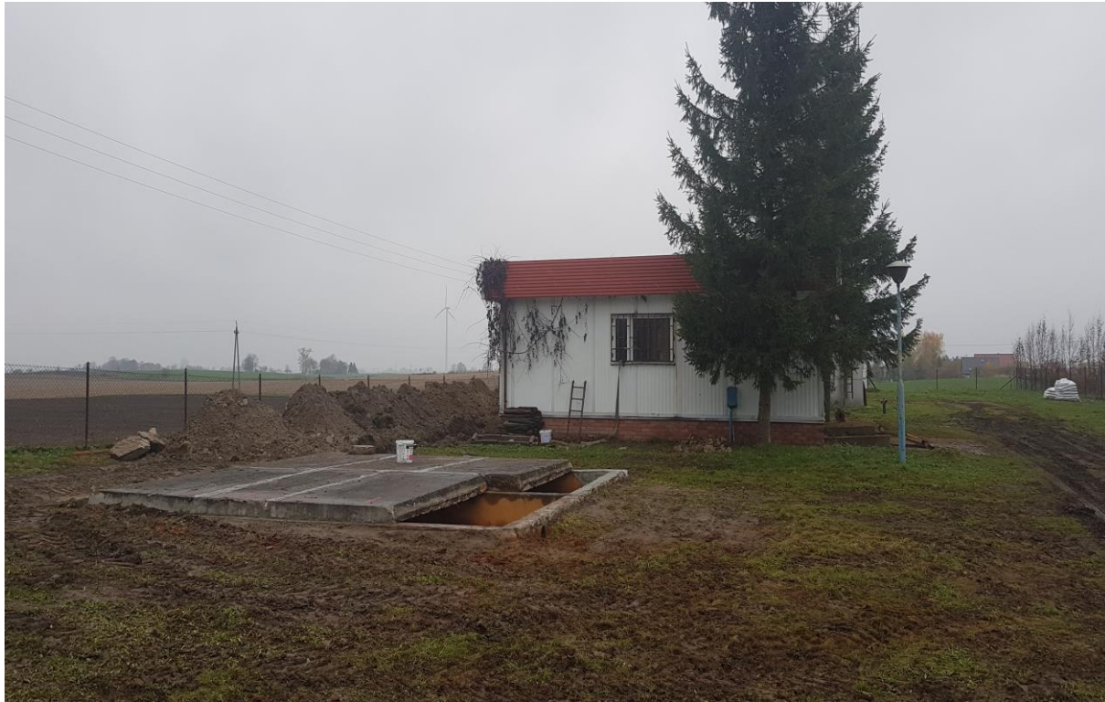
Remont SUW Lisewo
