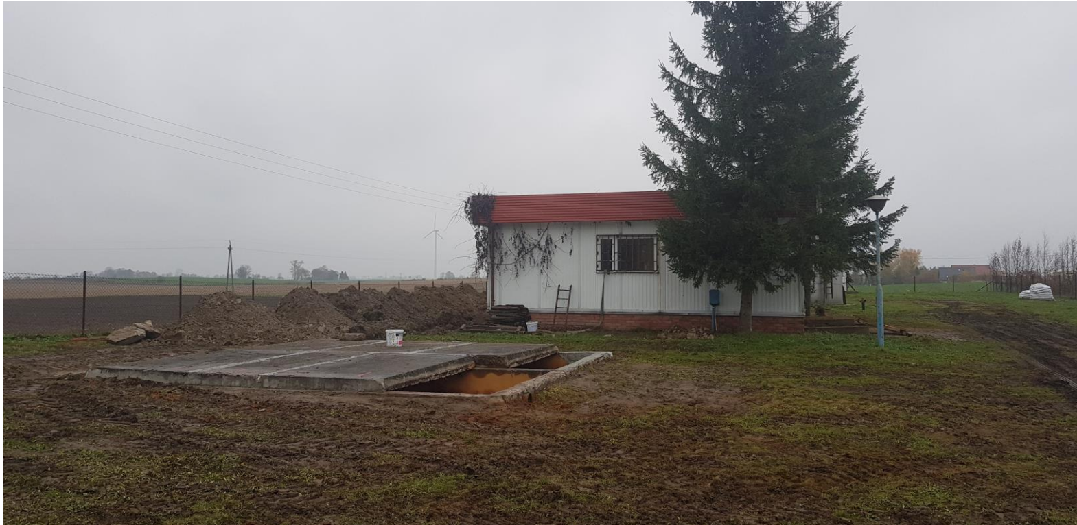
Remont SUW Lisewo
